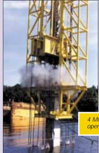
Port of Lake Charles in Louisiana, USA. The piles were 600mm (24in) square conthis second site three test piles were 600mm (24in) square concrete piles and an additional three piles were 750mm (30in) square concrete piles, driven in similar conditions
